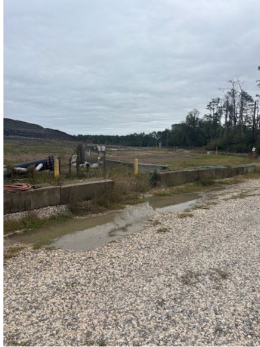
Photo 7 Southwest Corner Looking East
