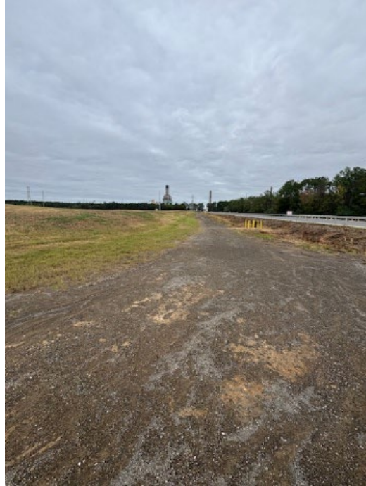
Photo 9 Southeast Corner Looking North
