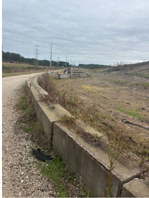
Photo 5 Northwest Corner Looking East
