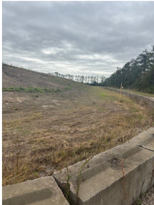
Photo 4 Northwest Corner Looking South
