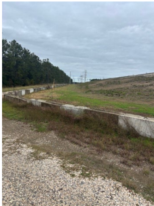
Photo 6 Southwest Corner Looking North
